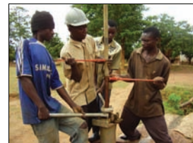
Image 1. Repair crew returns pump works fine well in Yonge, Zambia
